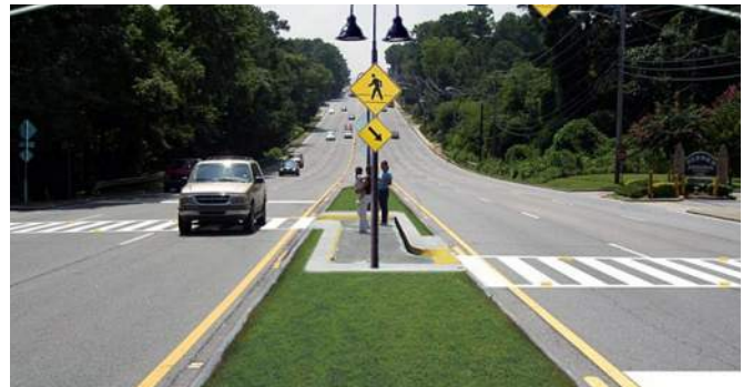
A pedestrian refuge island on a six lane roadway Source: www.harttma.com
