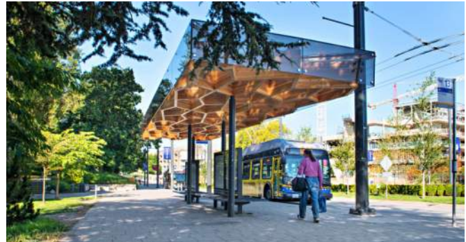
A placemaking bus stop in Vancouver, British Columbia (CA)
