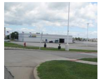
Sidewalk abruptly ends on Broadway near 84th Avenue
