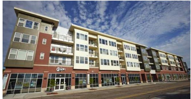
Mixed-use building with apartments and retail in Columbus, Indiana
