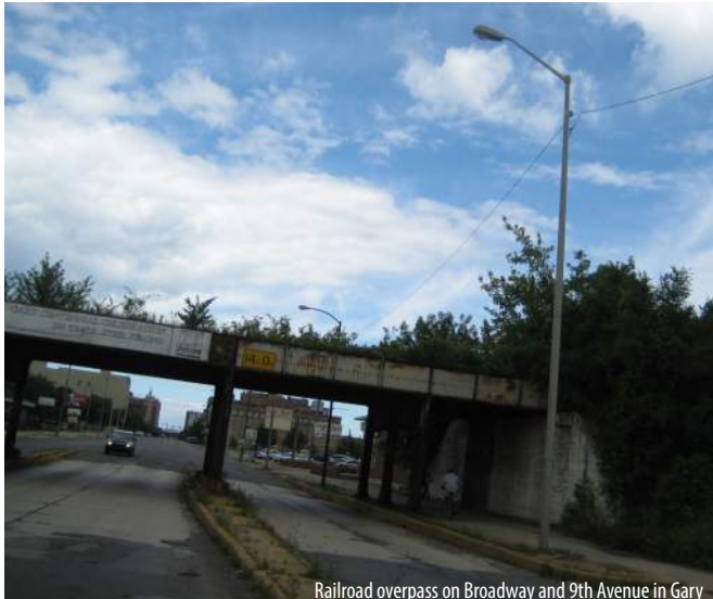
Railroad overpass on Broadway and 9th Avenue in Gary
